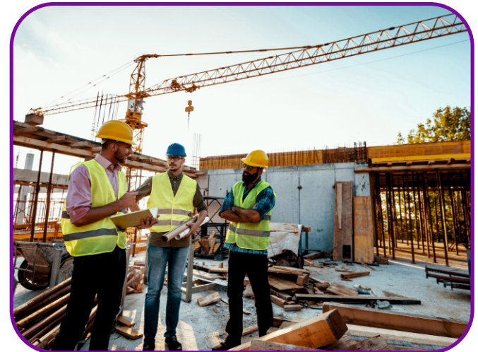
All type Construction Service
